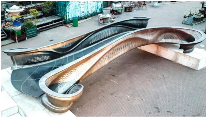
Fig. 3. WAAM - created bridge, [6]
